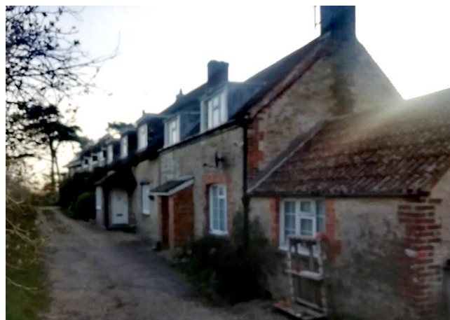
Figure 3: Cottages in Butter Street, Fleet
