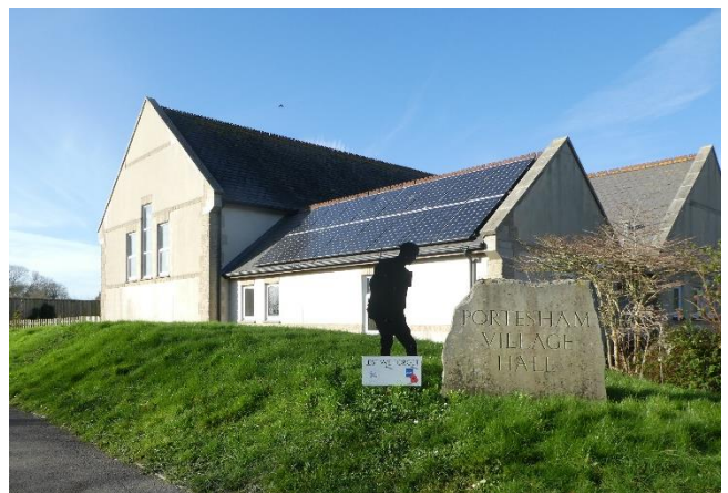
Figure 17: Portesham Village Hall
